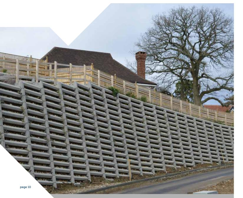
The Permacrib walls are up to 5.0m in height and various angle changes employed, highlighting the flexibility of the Permacrib system.
