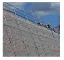
We will design Textomur with a slope angle up to 70°, but will recommend the use of gabion style finish to the front face. This is because the chance of long term growth diminishes the steeper the slope becomes. Where we are installing a stone faced finish, we will galvanise the Textomur cages and use a mesh with smaller aperture size. This has the added benefit of providing a maintenance free solution.
